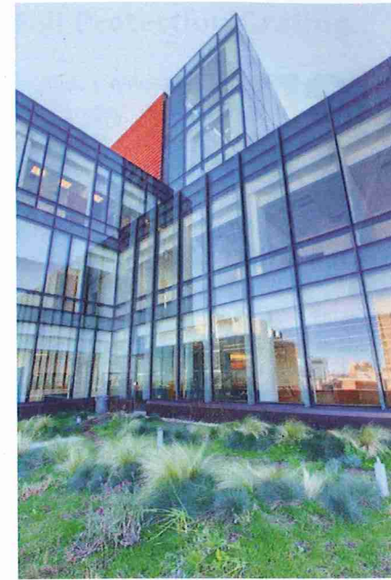
■ Recent projects include the garden roofs atop the Dana-Farber Cancer Institute, a 15-story building with multiple roof levels. Photo courtesy of Paradigm Partners.
