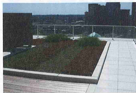
■ Marshall Roofing & Sheet Metal has carved out a niche for vegetative roof systems. Pictured is a vegetative roof at the Clarendon Condominiums. Photo by Alessandra Marshall.
